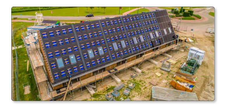
For more than 10 years, **GSE Intégration** has been developing an IN-ROOF mounting system that allows the construction of a solar roof with standard photovoltaic modules.
